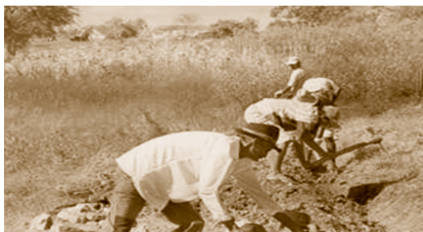
Figure 4 – Iguaçú farmers constructing a stone barrier
